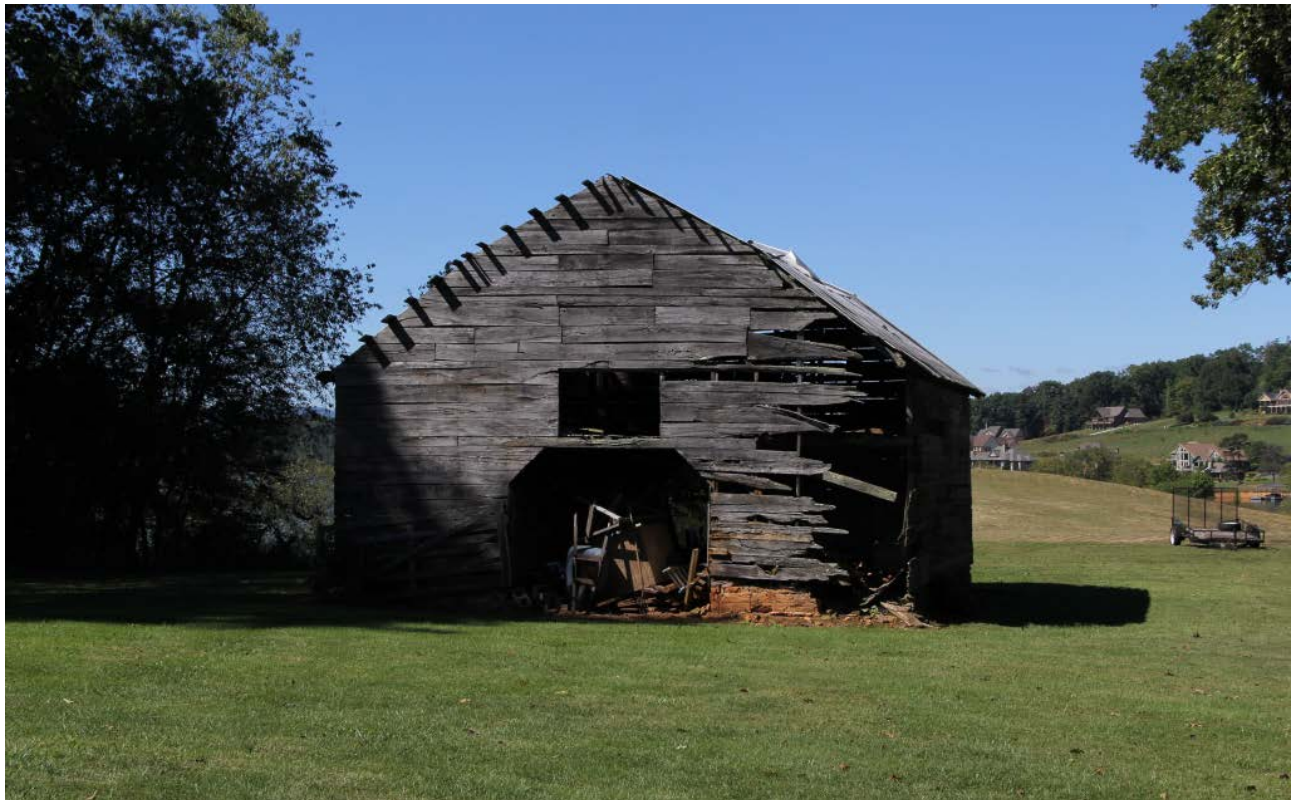
Barn, façade, view to west
