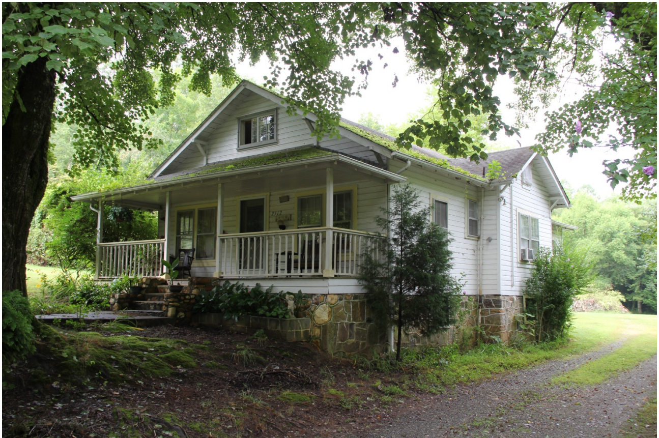
West House, 2112 Myers Chapel Road, view to southwest
