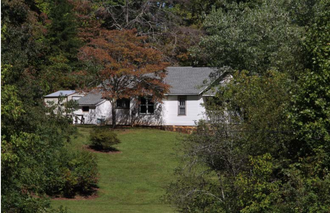
House, 2796 NC 175, view to northwest
