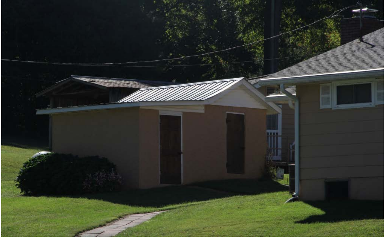
Shed #1, oblique front view to southeast
