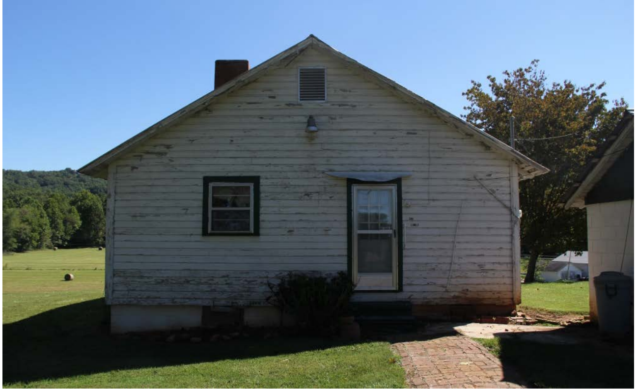
Hollifield-Eller House, rear elevation, view to east
