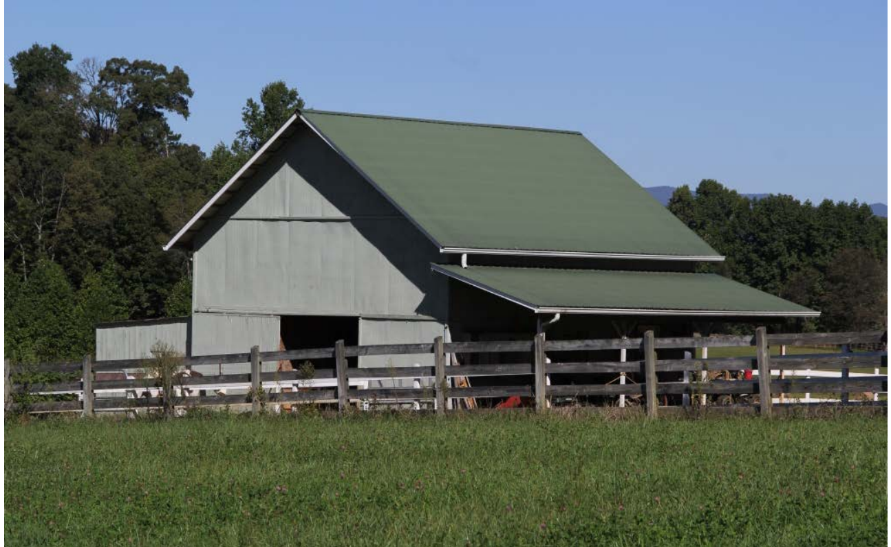
Barn, oblique view to northwest
