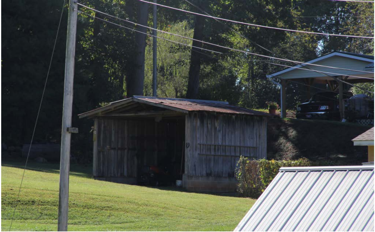
Tractor shed, oblique front view to southeast
