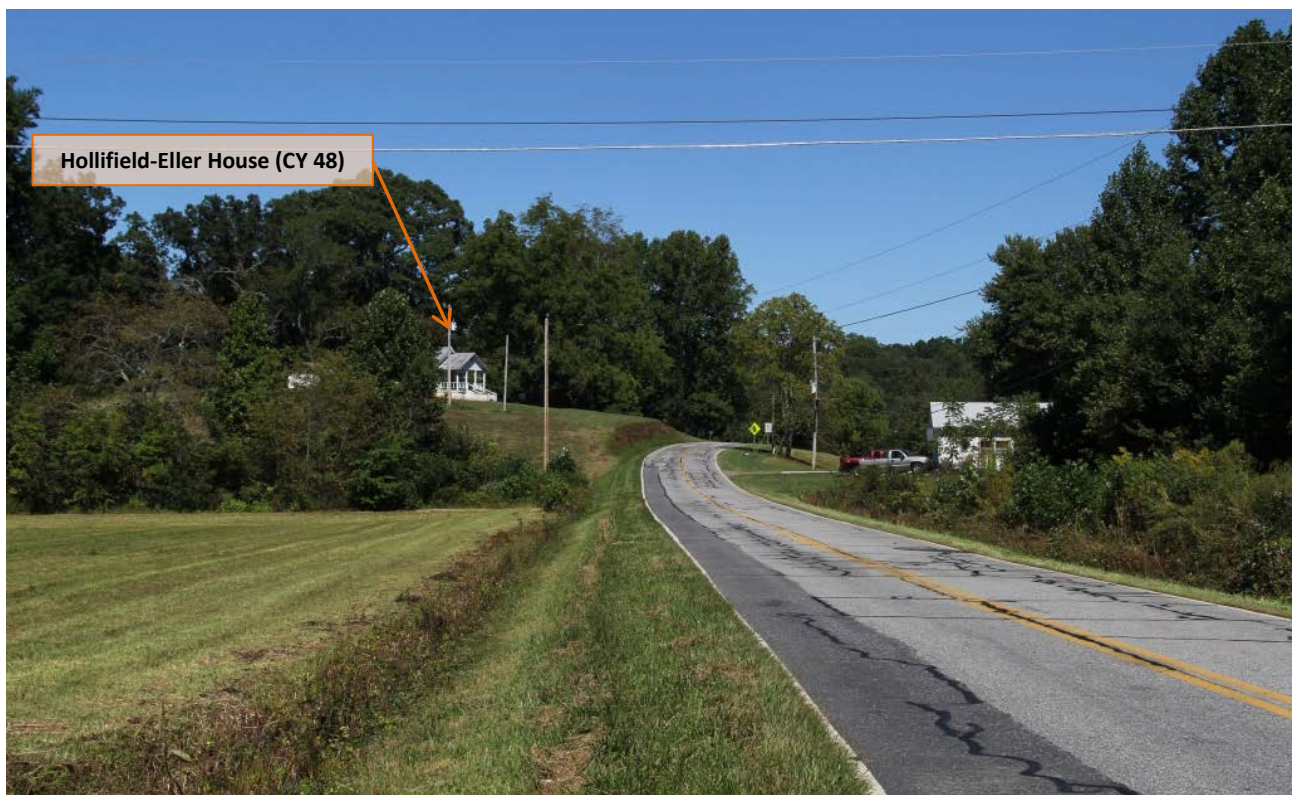
View north along NC 175 from Sneaking Creek Drive
