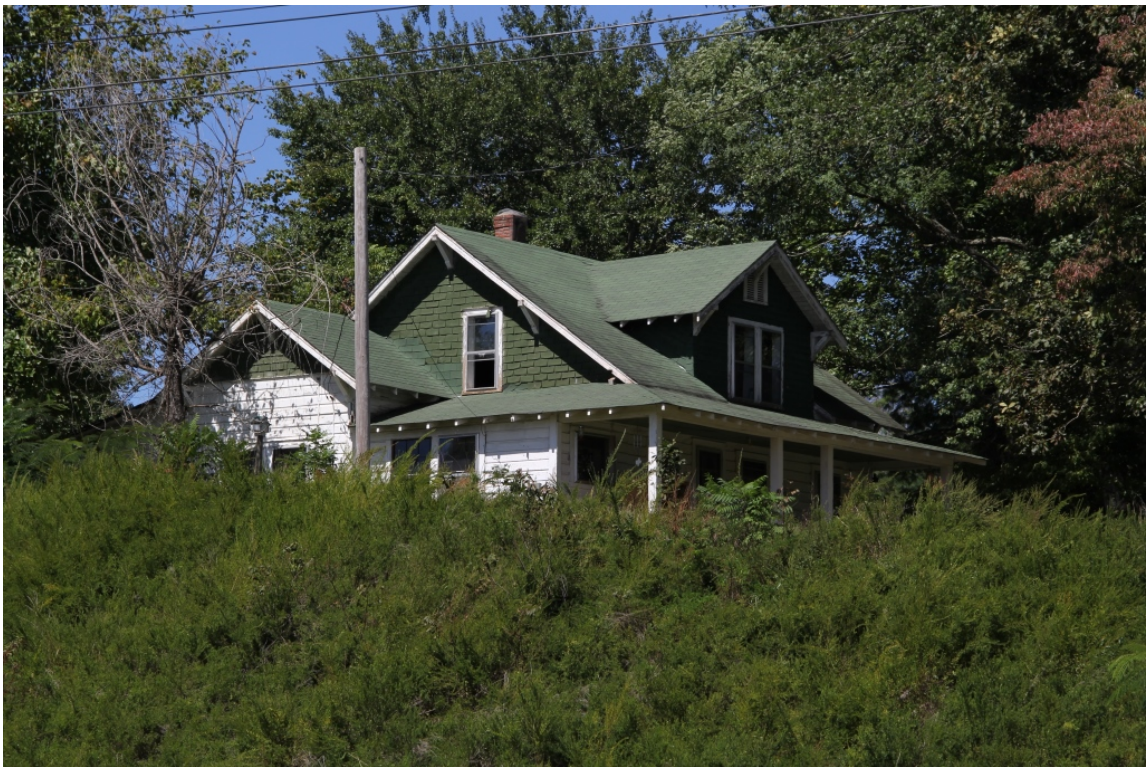
House, NW corner of US 64 and SR 1333, view to northwest
