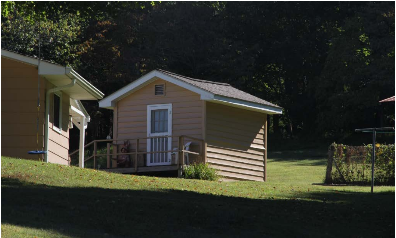
Shed #2, oblique front view to east
