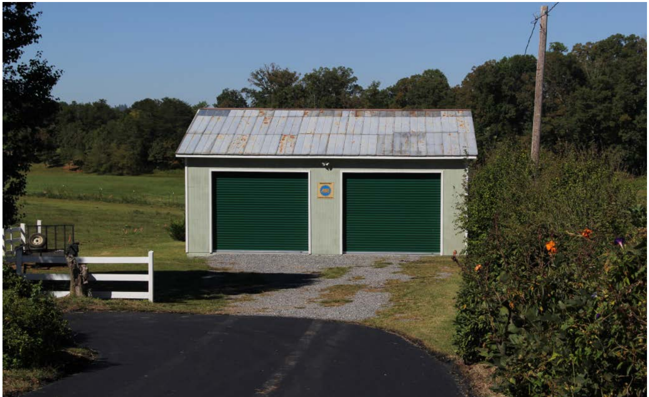
Garage, east elevation, view to west
